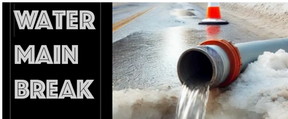
Image for a water main break
