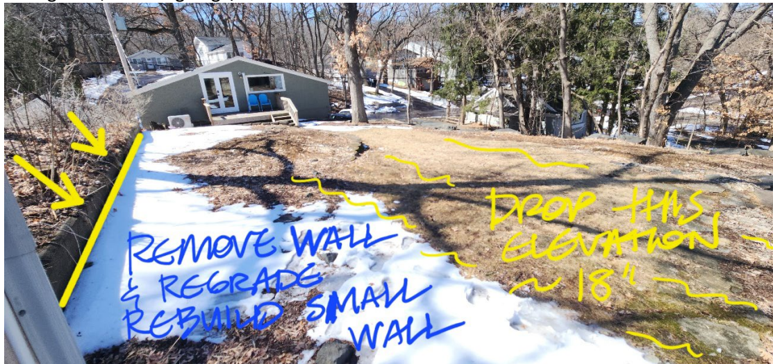
Facing south, toward 315 Wildwood vacant lot (panoramic view)
