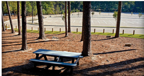
Figure 3. A large PICP parking lot manages an overall site slope of 12% using terraced areas.
