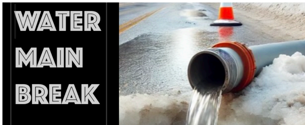
Image for a water main break
