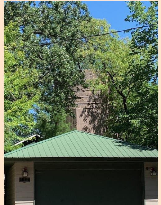
Hidden behind the foliage is the original 1920 water tower as seen in 2021. Photo courtesy of Scott Freeberg
