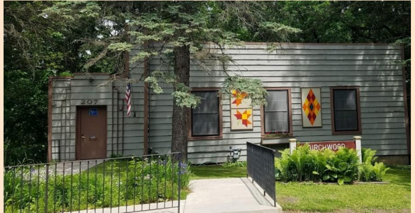
Birchwood City Hall prior to 2021 Renovation. Photo courtesy of Mary Wingfield
