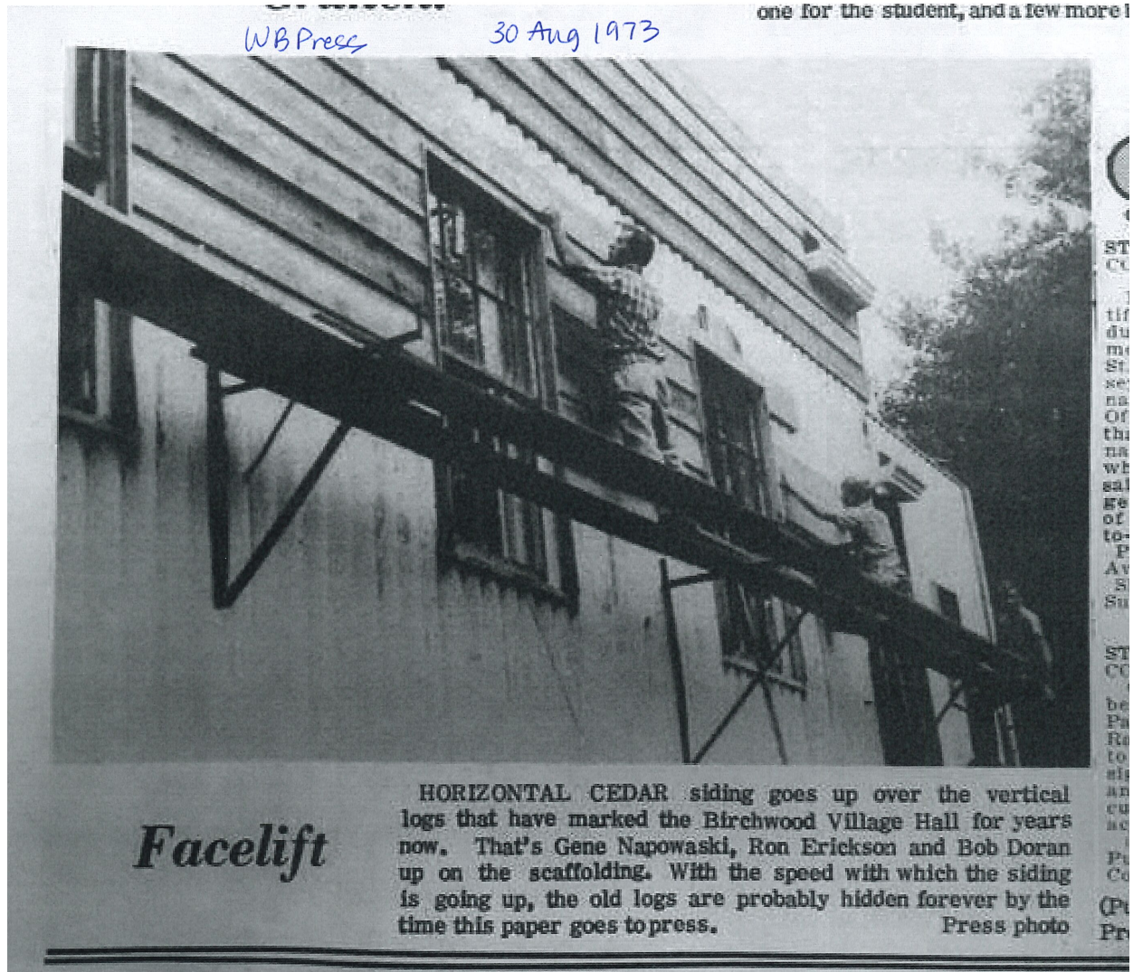
1973 clipping from the White Bear Press showing a crew installing horizontal cedar siding over the original log siding.
