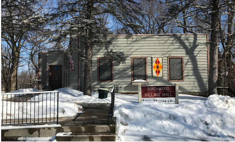
Primary elevation and entry. Note stepped massing at entryway and wooded setting. Shown from the parking lot.
