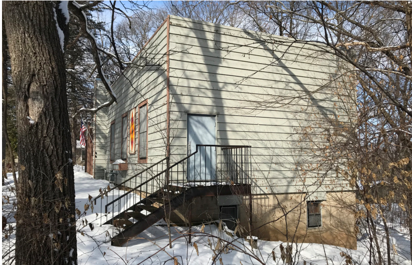
Southeast elevation, showing sloping site and original CMU foundation.
