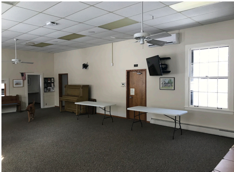
Main assembly room looking at northeast wall. The window opening shown is believed to be an original opening. Two others were removed when the addition was built. Note doors to Storage/AV Room and Restroom, both added in the 1980s.
