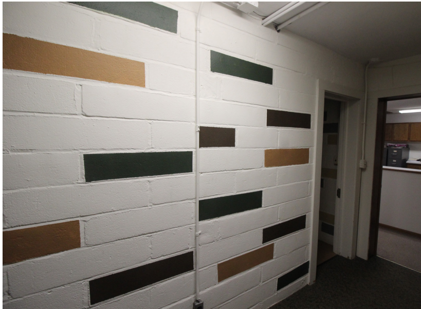
Original CMU foundation walls visible on lower level.
