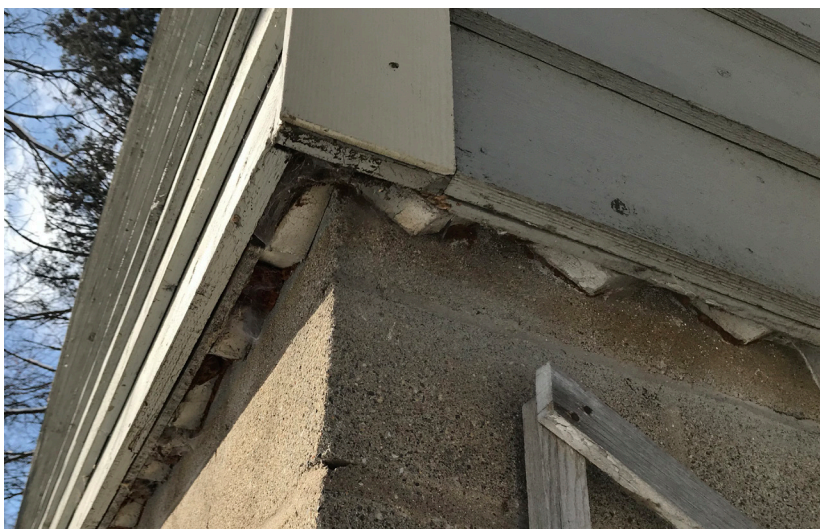
Evidence of original half-round log siding is visible beneath the horizontal cedar siding added in the 1970s.
