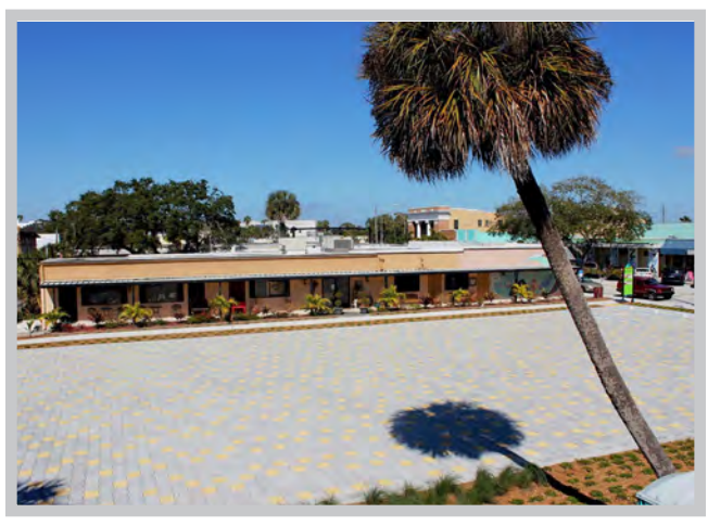
Completed job City of Melbourne
