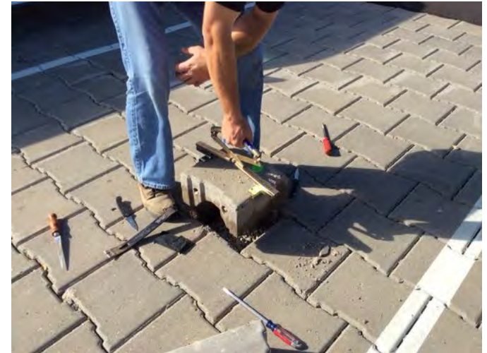
The PaveDrain System can be mechanically lifted for more thorough cleaning.
