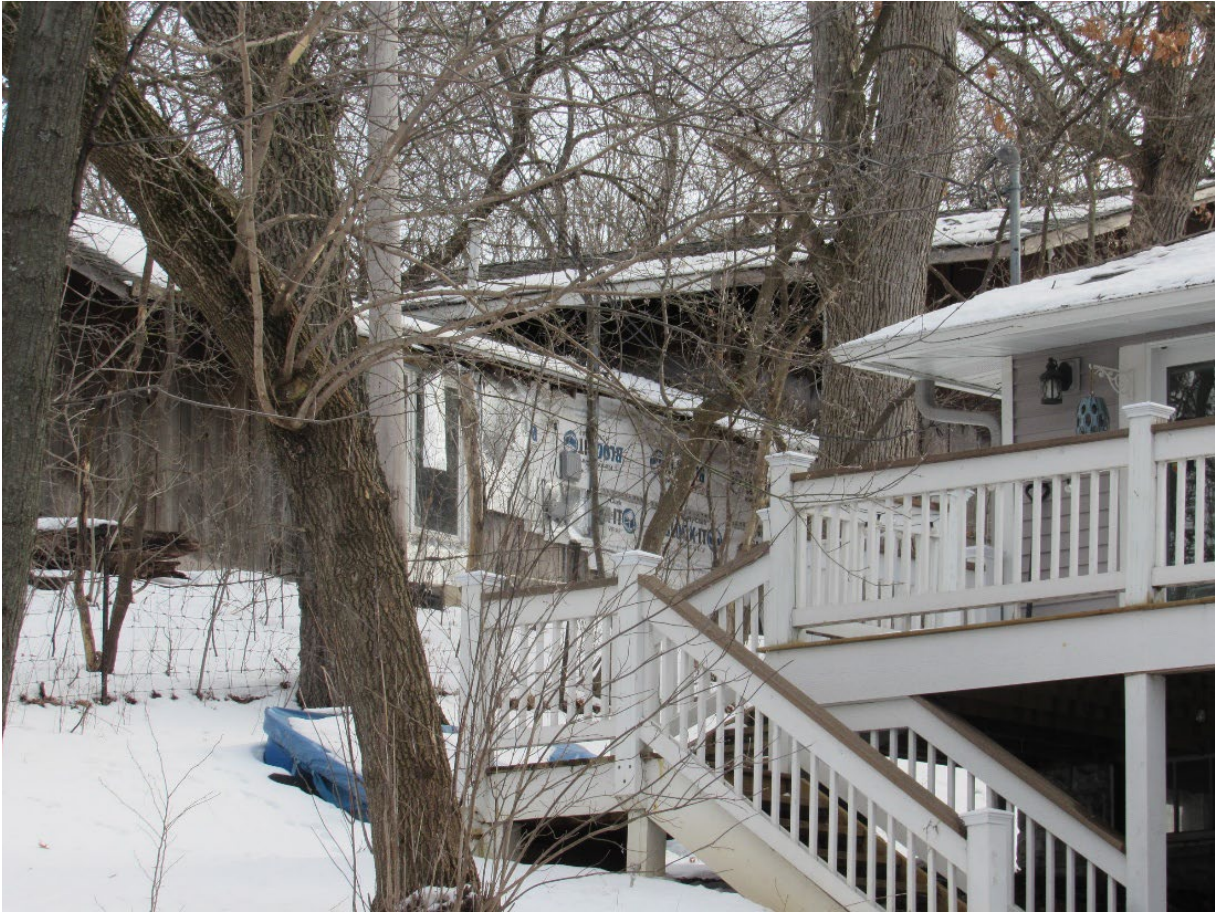
House wrap on west side of 310 (3/29/2024):
