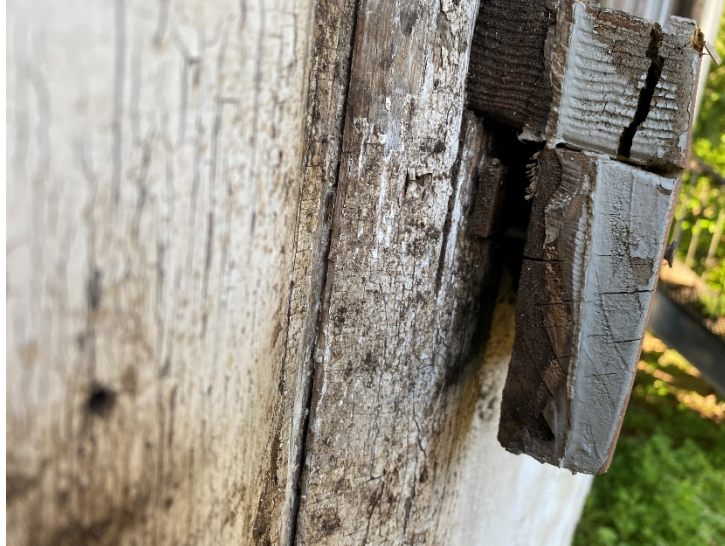
Figure 2 Photo shows the end of a decayed and split window sill and the poorly fit apron under the sill.
